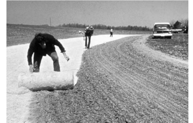
Exposed soils are very vulnerable to erosion. Mulch or other ground cover protects surfaces from wind and storm water erosion, as well as allowing vegetative growth.
