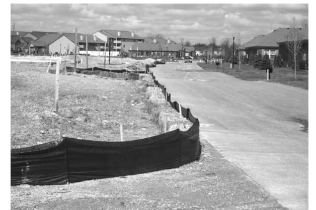
Silt fences prevent the offsite transport of sediment at construction sites.
