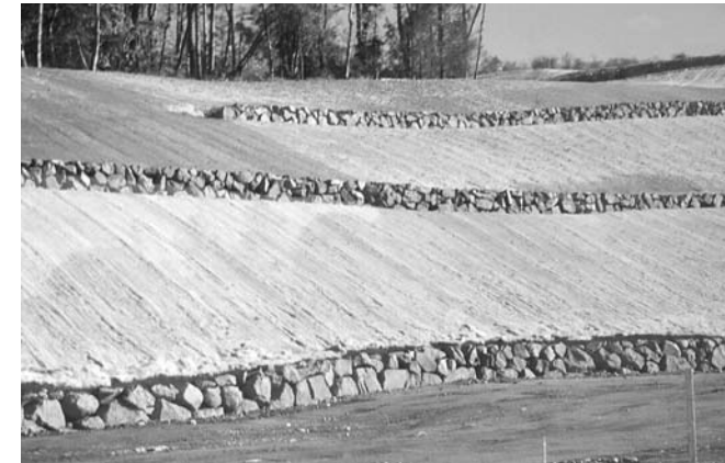
Terracing can be used to slow runoff. Lined diversion ditches direct flow away from exposed areas toward stable portions of the site.
